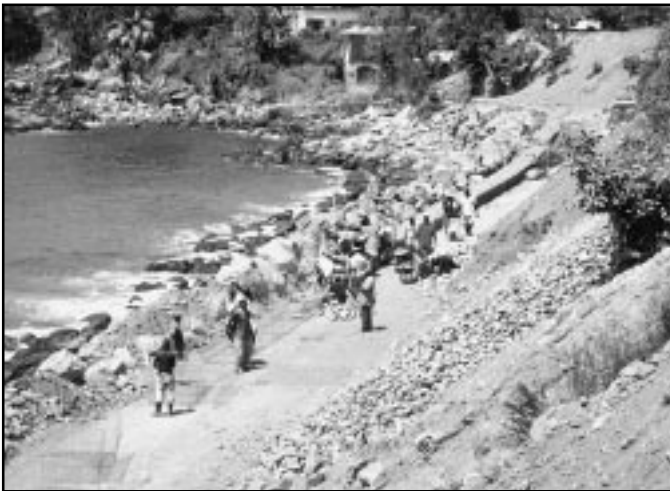
Hillside retaining wall being built
