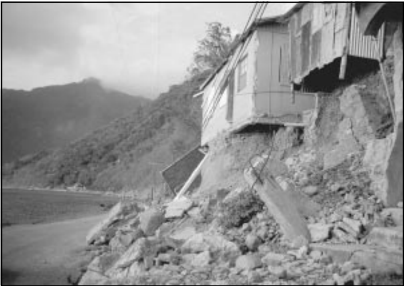
Storm surge damage – Hurrican Lenny
