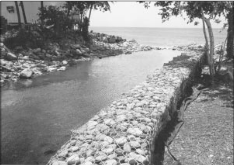
Gabion to reinforce stream bank
